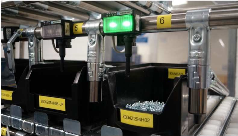
Picture 1: The new Guided Operator Solutions from Mitsubishi Electric are used to increase quality by eliminating mistakes during manual parts picking process.
