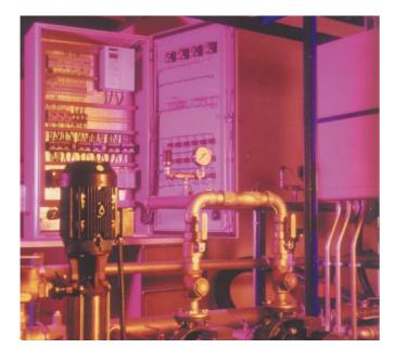
On the new system designed and built by recycling equipment specialist K A Wing, a Mitsubishi Freqrol A140E 7.5kW inverter drives 2 pumps which deliver water into the shredder via a unique injection system. The amount of water injected is precisely matched to the activity of the shredder's 3.7MW drive. K A Wing specified the Freqrol inverter with PI control as an internal option, so that the inverter automatically maintains water pressure by varying the pumping effort to match demand.
